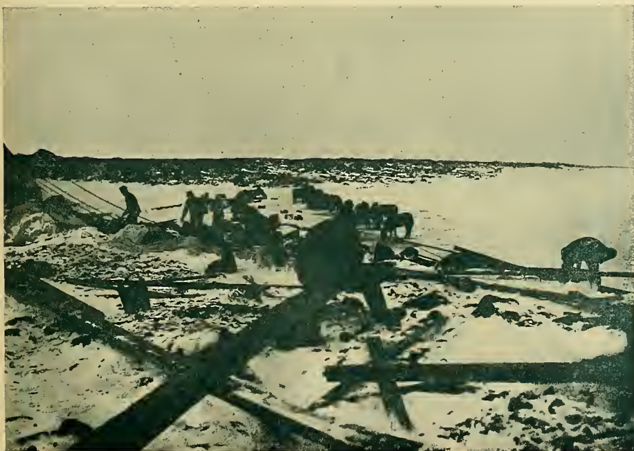
WE START TO BUILD OUR WINTER QUARTERS
